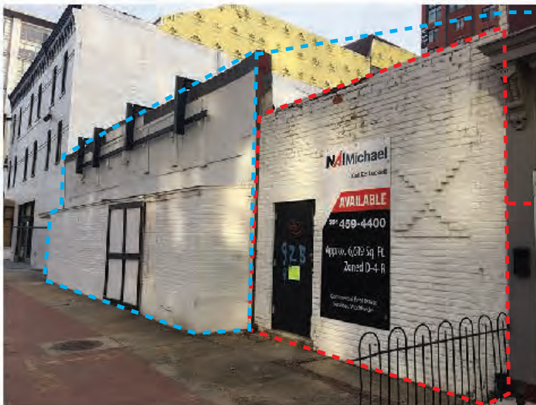
EXISTING BRICK FACADES
