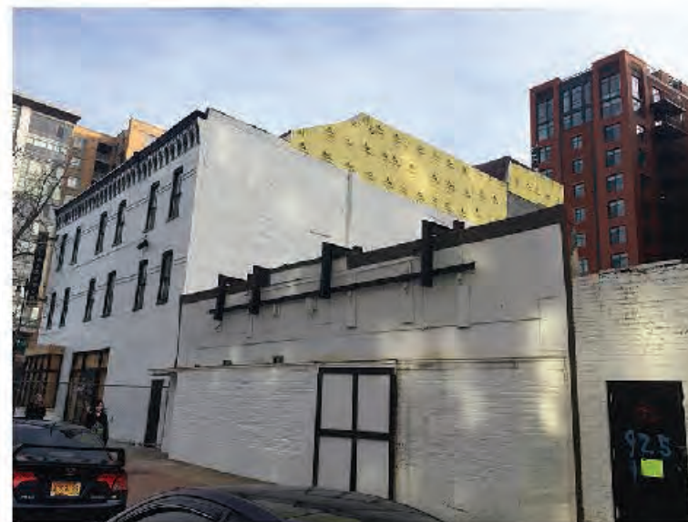
EXISTING BRICK FACADES
