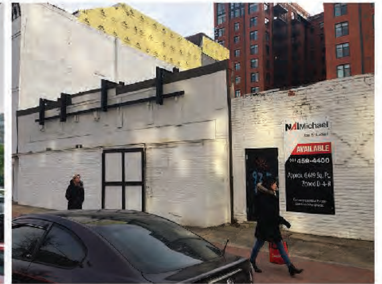
EXISTING BRICK FACADES
